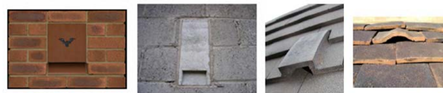
examples of bat tiles, bricks, integrated bat boxes from BCT http://www.bats.org.uk/pages/bat_boxes.html
